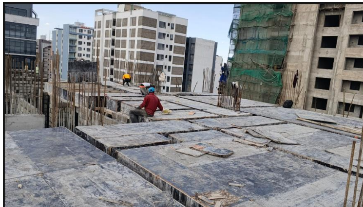
Shutter works across the floor
