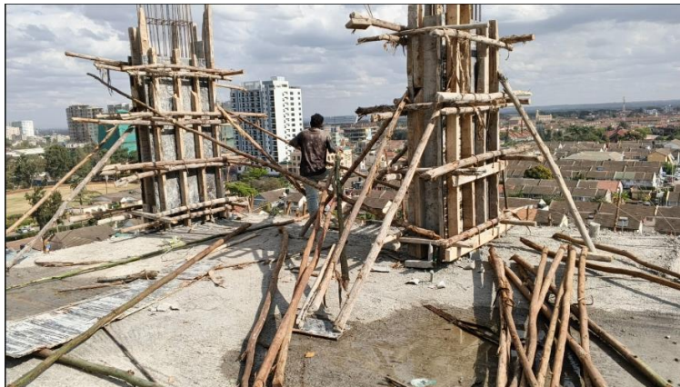
Column casing 11th–12th
