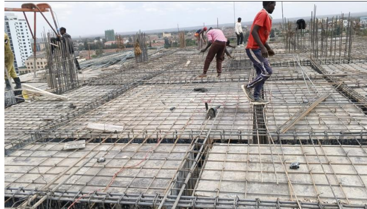
Beams and slab reinforcement
