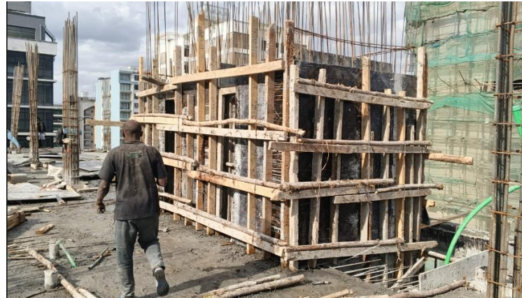
Lift-shaft formwork
