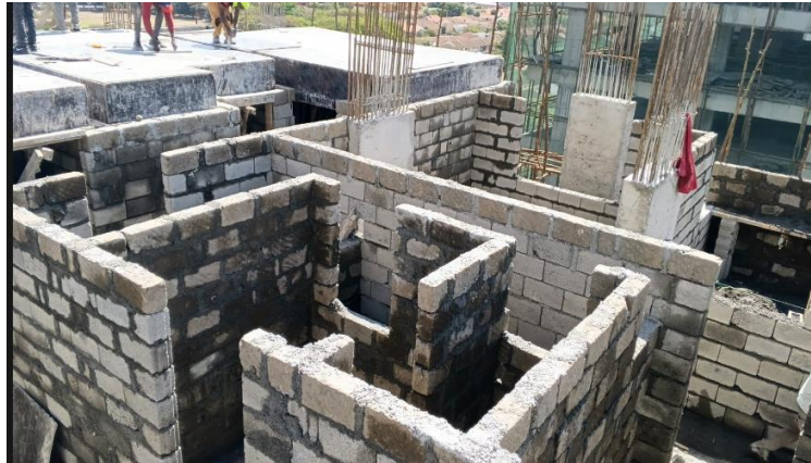
Internal partitions rising
