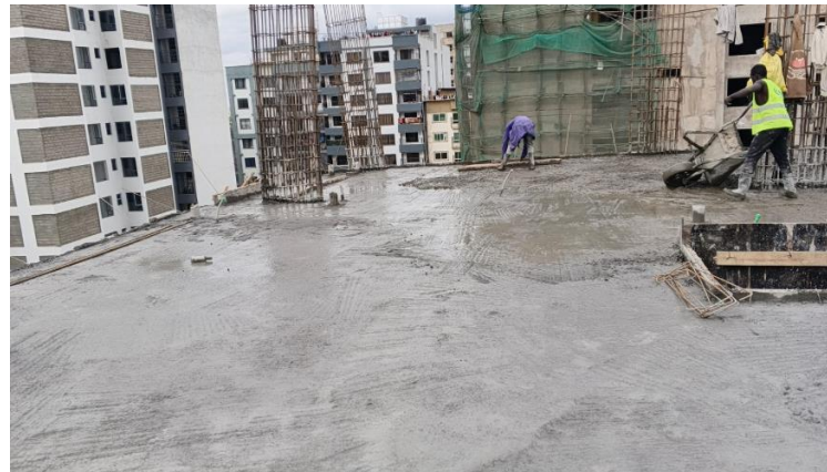
11th floor slab casting
