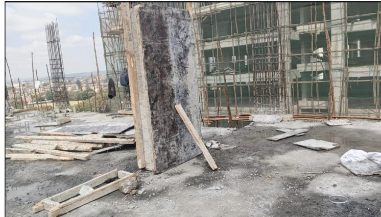
Column casing 10th–11th
