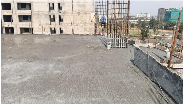
10th floor suspended slab casting
