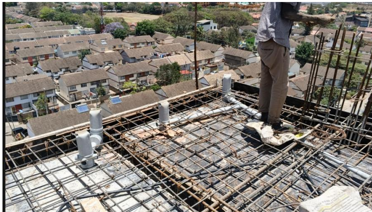
MEP works in the slab
