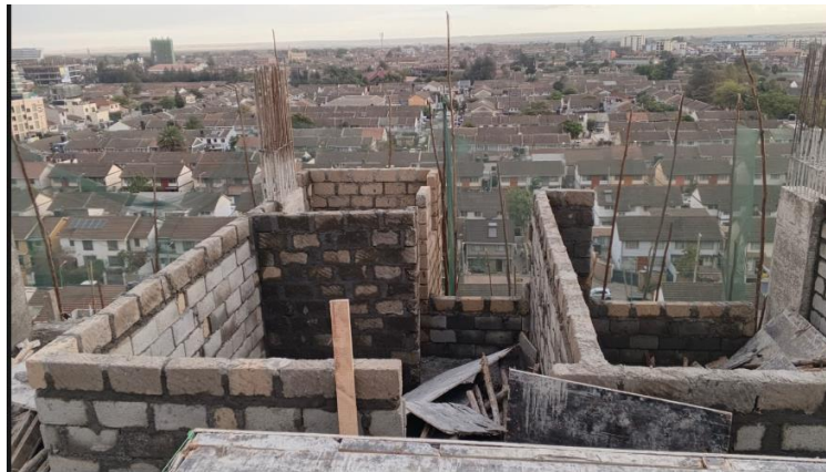
Walling progressing across the floor
