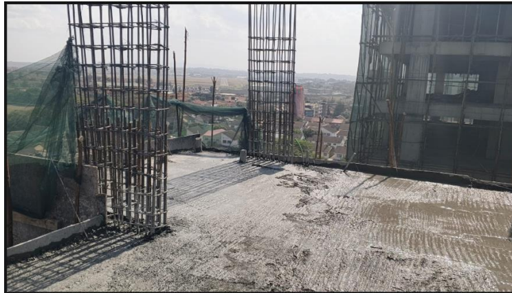
Slab cast, column starter bars visible
