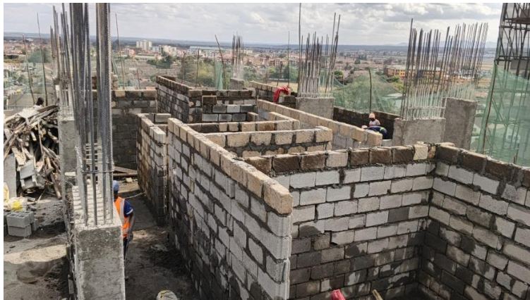
External & internal walling
