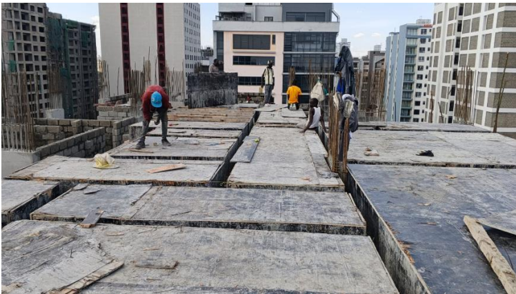
12th floor suspended slab shutter
