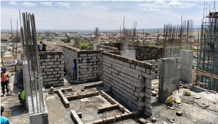
11th floor external & internal walling
